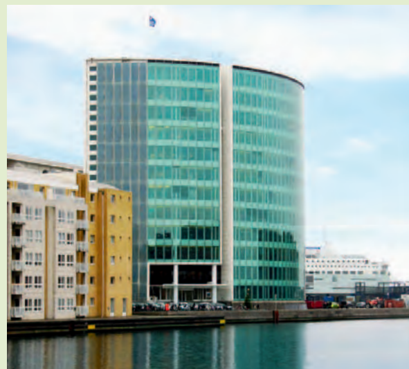
The new façade at ALM Brand Headquarters in Copenhagen.
